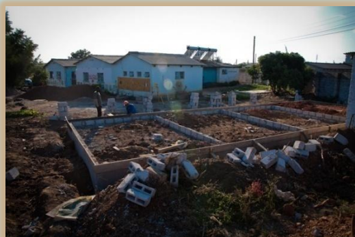
Beginning of the construction works.
